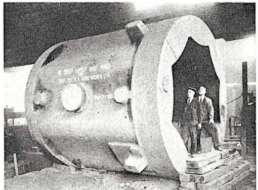
Weighing over 150 tons, 13½ feet long and 12 feet in diameter, this ingot mold is said to be the largest in the world. It constituted the biggest single load ever hauled by rail in England and necessitated special rating of freight train.
