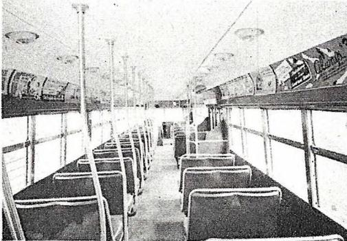
Top—Exterior view of the new electric car developed by Electric Railway Presidents' Conference Committee. They start and stop quicker, can speed at 50 m.p.h., and are fitted with three brakes—dynamic, magnetic and air. Bottom—Interior view of the car showing the seating arrangement
