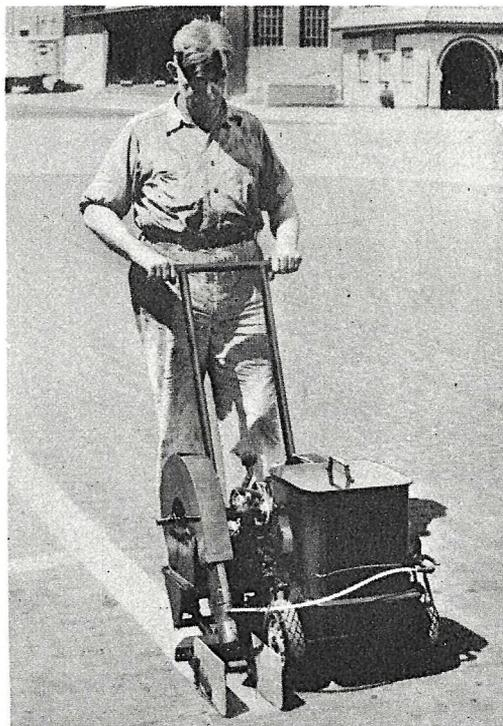
Powered by a  $\frac{3}{4}$  horsepower gasoline engine, this traffic line marker is operated by one man. Paint from the nozzle is sprayed onto the pavement by means of a powerful fan.
