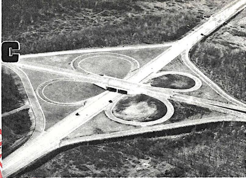
A "Cloverleaf" type highway at Paramus, N. J. keeps up with automobile age. With super roadways crossing, safety is assured by this Limited Way.
