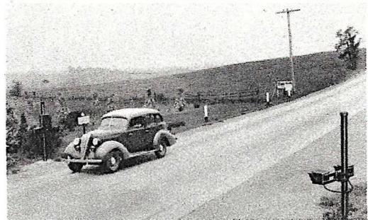
Placed along a highway so passing autos intercept its light beams, this device automatically counts each car and prints a total once every hour. Passing pedestrians do not effect it.
